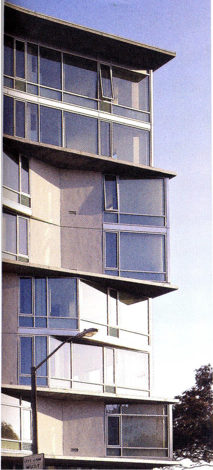
Parkview Terraces, San Francisco, 2008 Architects: Kwan Henmi Architecture (architect), Fougeron Architecture (consulting architect) Owner/Developer: A.F. Evans and Chinatown Community Development Center Photography: Rien van Rijthoven
